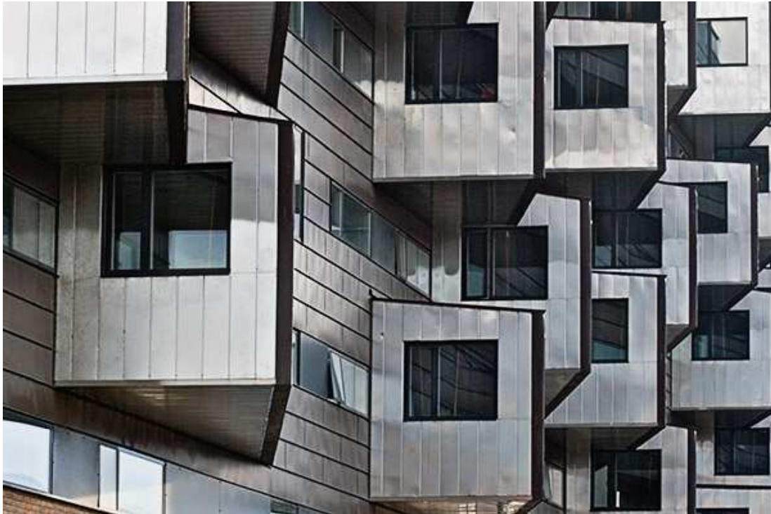
Figure 8.3 – Photo showing the projecting bays on the northern side of Pooley House student accommodation block, Queen Mary University.
